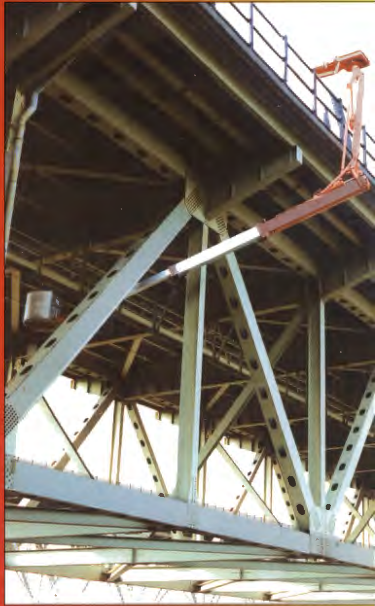
High bridge rails do not restrict Bridgemaster's below deck through-truss deployment.
