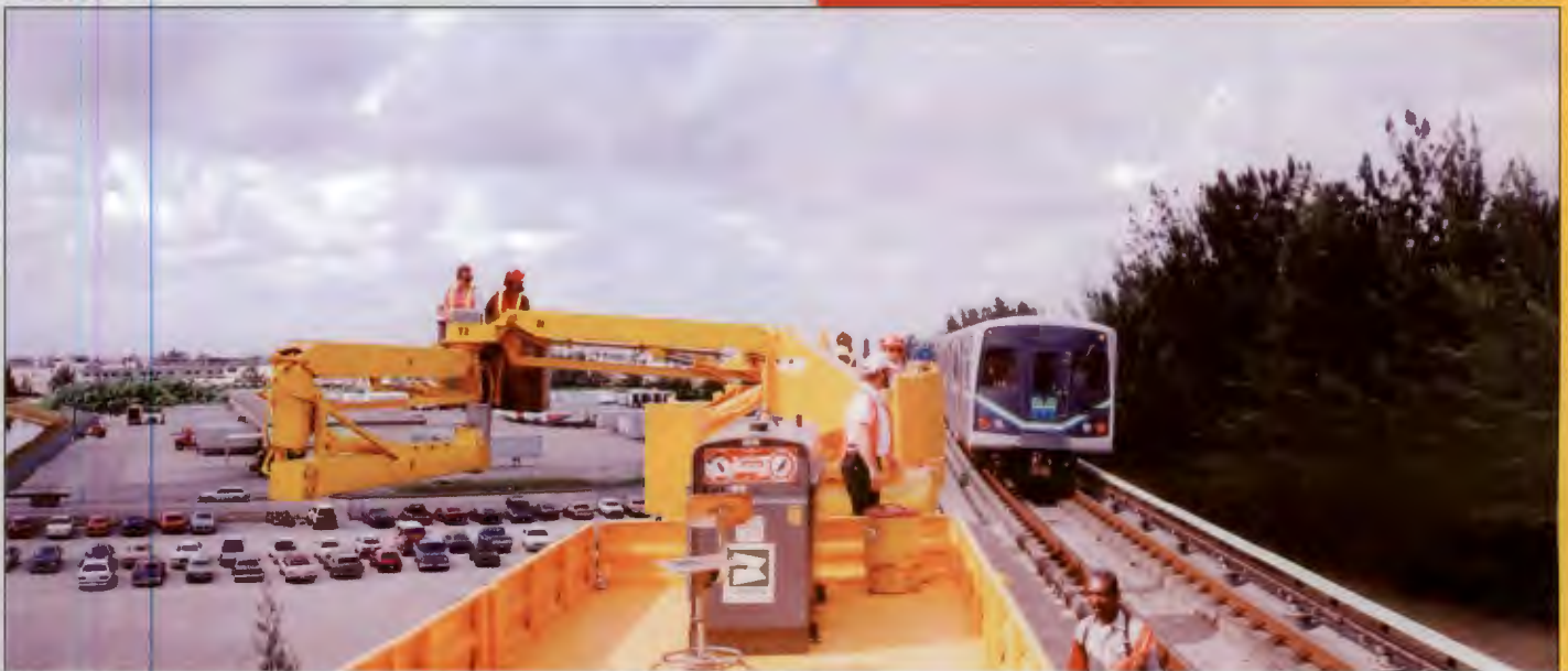
Bridgemaster Jr, flat-car mounted flagship unit heads a work-train-consist for inspection, repair and
