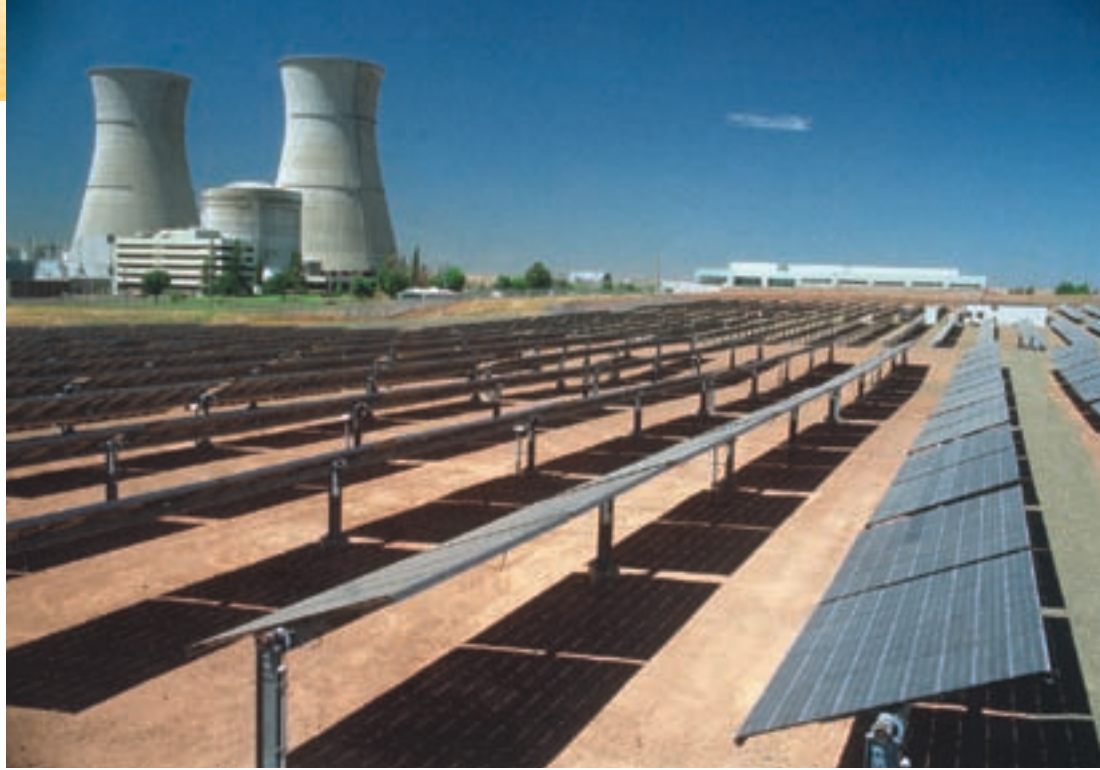
Gone but not forgotten: David Freeman helped put the Rancho Seco nuclear power facility in Northern California out of commission. Surrounding it is the alternative: a two-megawatt solar plant that powers 660 Sacramento homes.
