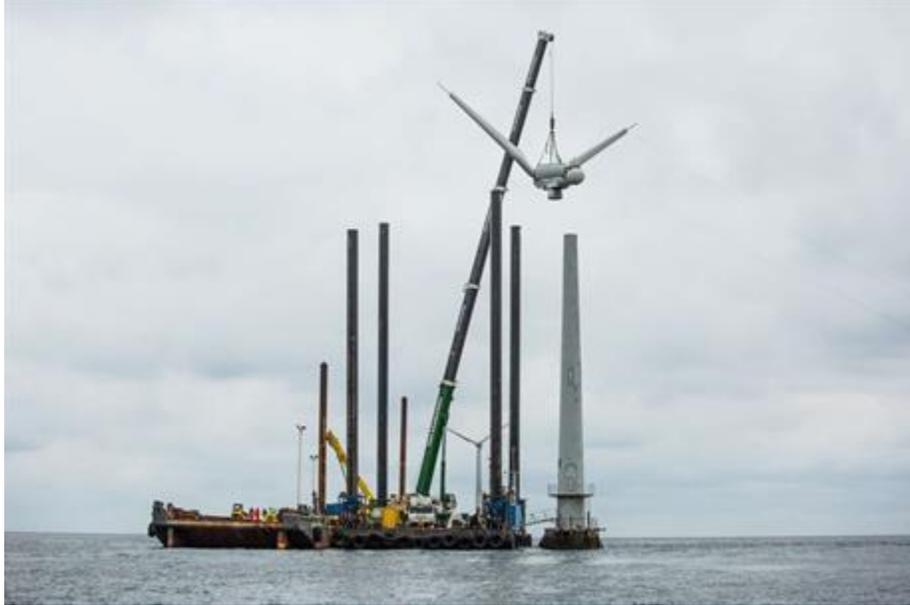
Decommissioning has started at the 26-year old Vindeby offshore project, one of the world's first The 4.95MW Vindeby offshore project was installed in 1991 using 11 Bonus 450kW turbines. It operated 1.5-3.0km off the southern Danish coast.
