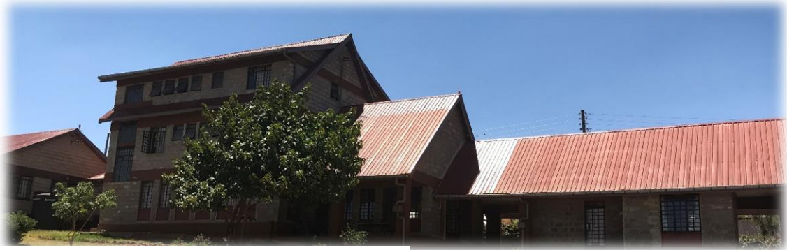
Ahadi houses for boys, staff and office after repainting trim
