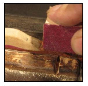
**Step 37:** Use a miniature sanding block, and a small piece of 150 grit paper to sand off any glue remnants from the bottom of the molding. This step will make it easier to form a well made collar when the new glue is applied.
