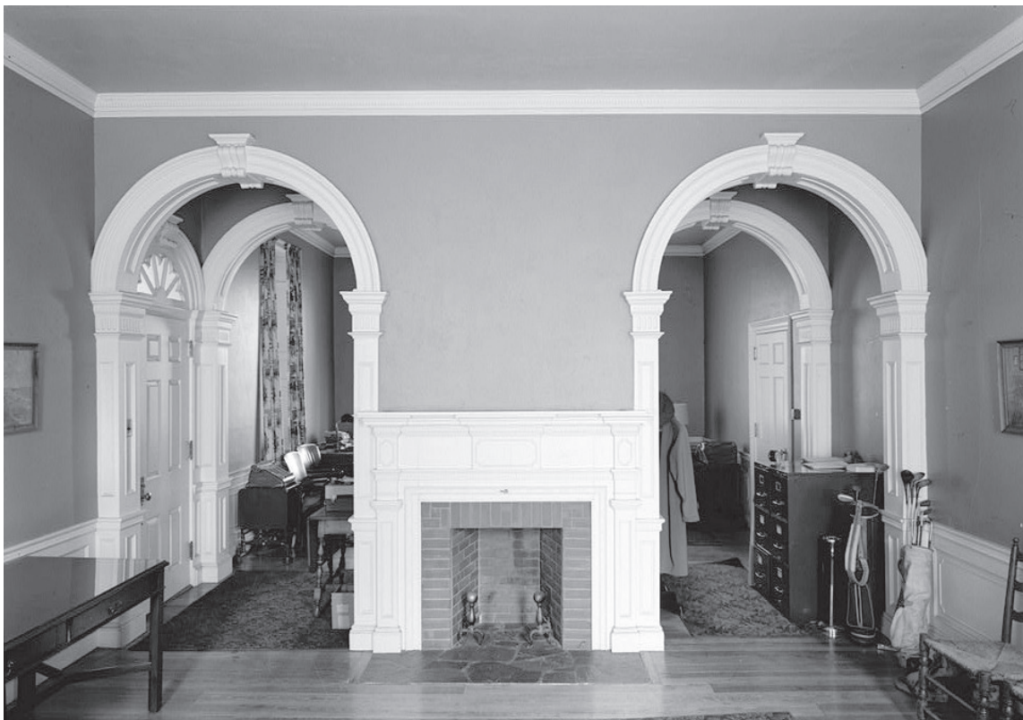
September, 1958 NORTH WALL OF WEST END
