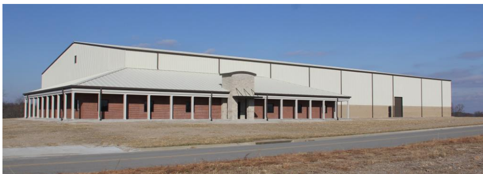
Eastern Kentucky Business Park Spec Building
