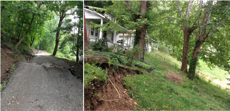
Figure 5. Large landslide complex in Paintsville, Johnson County. This landslide damaged several homes and two streets in the area.
