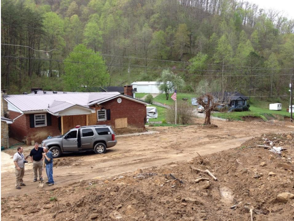
Figure 6. Distal toe of a damaging debris flow, Floyd County. The debris flow severely damaged a home and covered the road with debris.
