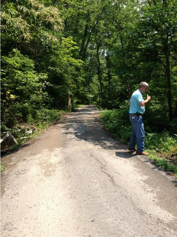
Figure 10. Landslide that has displaced and damaged a road, Pike County.
