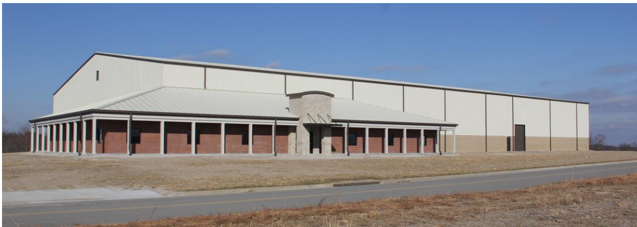
Eastern Kentucky Business Park Spec Building
