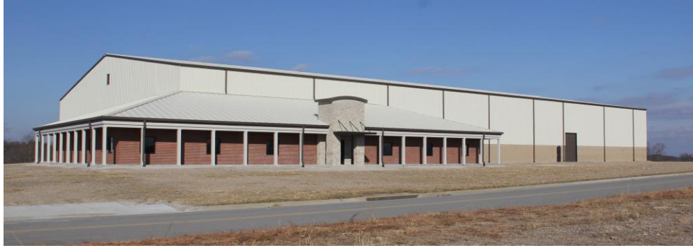
Eastern Kentucky Business Park Spec Building
