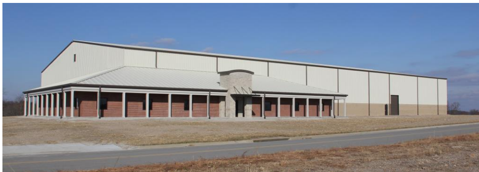
Eastern Kentucky Business Park Spec Building
