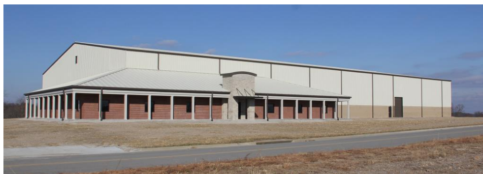
Eastern Kentucky Business Park Spec Building
