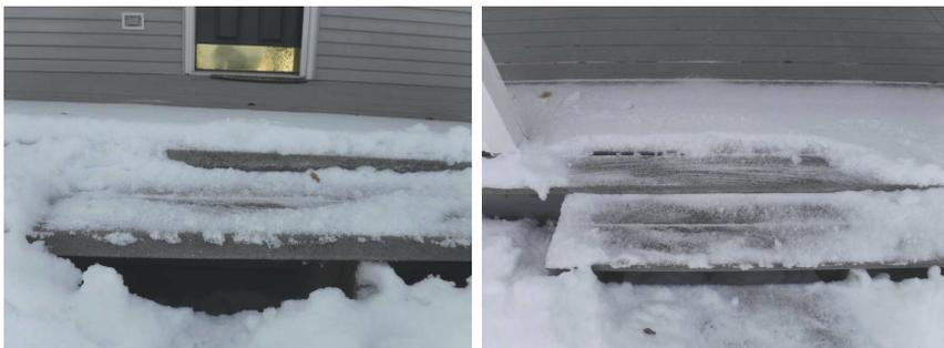
Stair tread and decking should be at the same elevation or an equal rise between all stair risers. A potential tripping safety concern.
