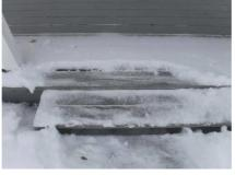
Stair tread and decking should be at the same elevation or an equal rise between all stair risers. A potential tripping safety concern.
