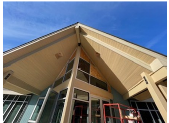
The entrance roof is complete.
