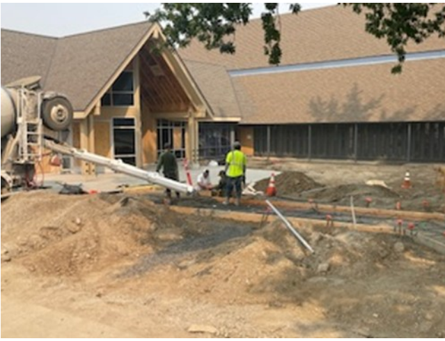
New sidewalks are formed along the front entrance.
