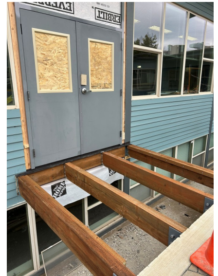
Walls are reinforced in preparation for the patio bridge and a new doorway to Fellowship Hall.
