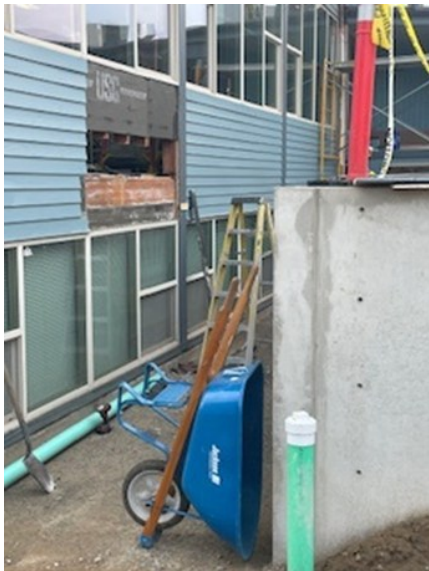
Walls are reinforced in preparation for the patio bridge and a new doorway to Fellowship Hall.
