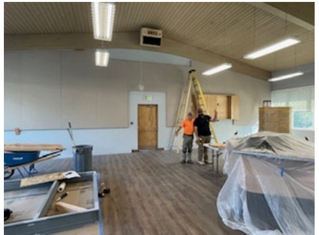
Edgar and Nate put the finishing touches on acoustical tiles in the Fellowship Hall.
