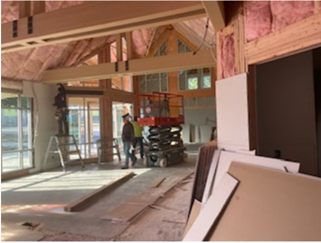
The narthex gets insulation and drywall.
