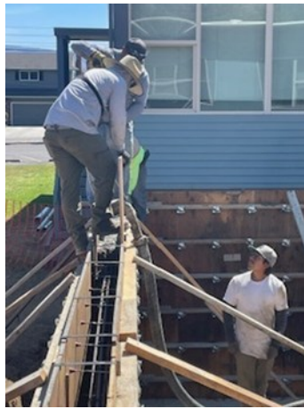
A retaining wall goes up for the back patio space.
