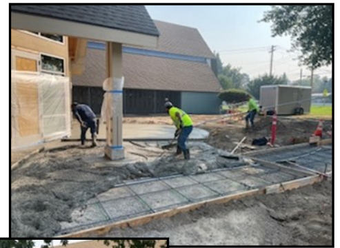
Pouring concrete around the new addition
