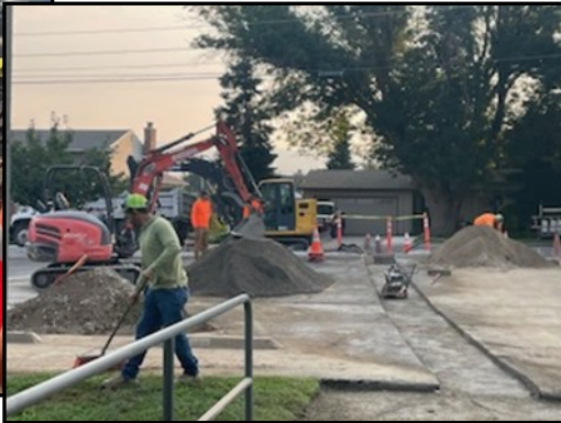
Creating a new water line to Elliott Street
