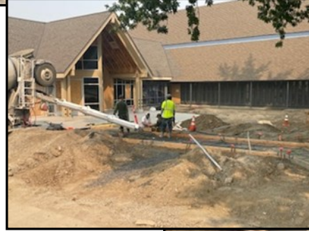
Pouring concrete around the new addition
