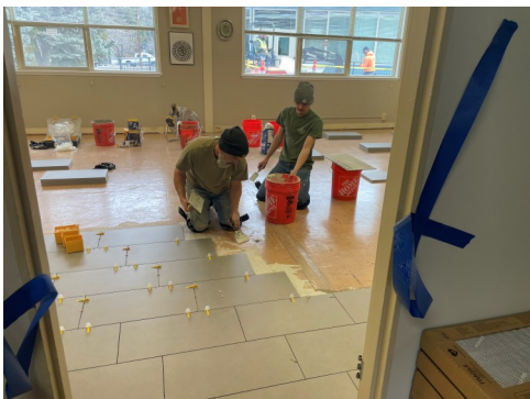
Sound-reflective tiles are laid in the Rehearsal Room. .
