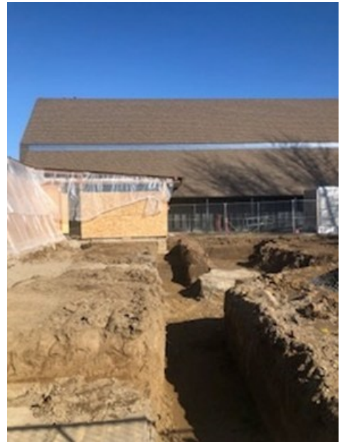
New foundation trenches dug
