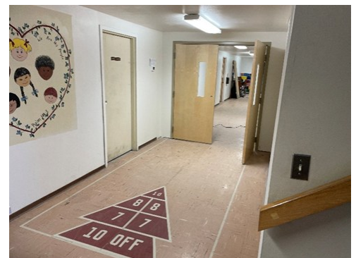
The basement floor's temporary wall is removed to reveal new fire doors.
