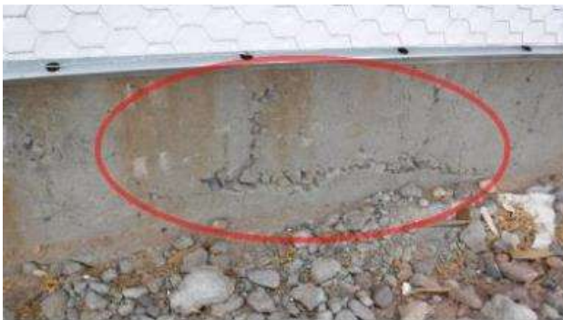
ROUGH SURFACES AND CHIPS AT FOUNDATION.
