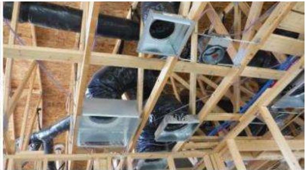
LAUNDRY BOX NOT FULLY SECURED / SUPPLY AND RETURNS CLOSE TOGETHER.
