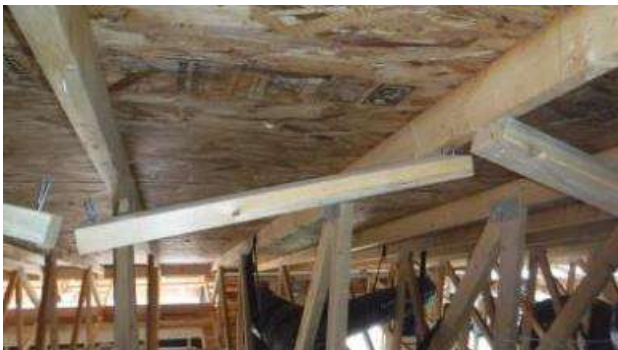
LOOSE TRUSS SPACERS IN ATTIC.
