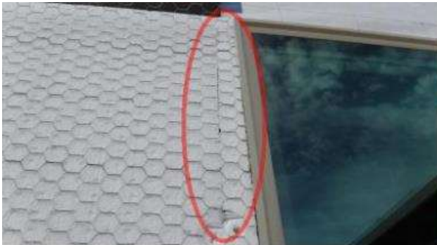
LATH SEAM NOT TAPED-SEALED / MISSING FASCIA CLIP.
