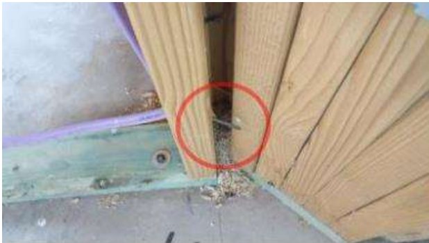
SHINERS AT WALL FRAMING / SEPARATIONS-UNEVEN FRAMING AT PATIO DOOR.
