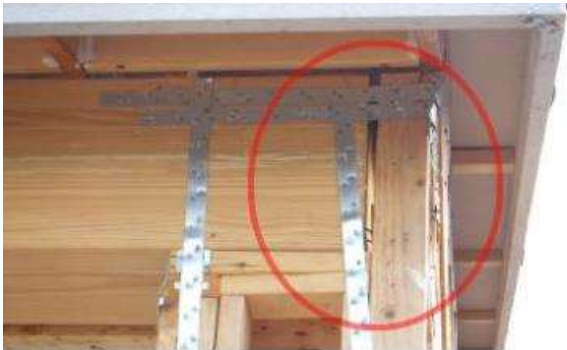
SEPARATIONS AT PATIO BEAM / POSSIBLE MOLD AT GARAGE HEADER.
