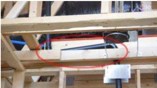
IMPROPER RISE AT VENT PIPE / WIRES NOT SECURED WITHIN 12"
