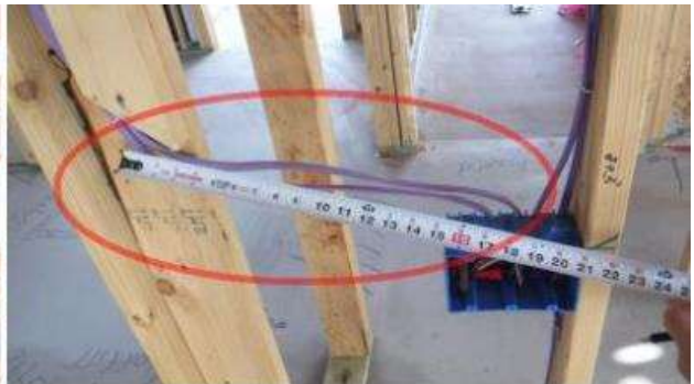
LAUNDRY BOX NOT FULLY SECURED / SUPPLY AND RETURNS CLOSE TOGETHER.
