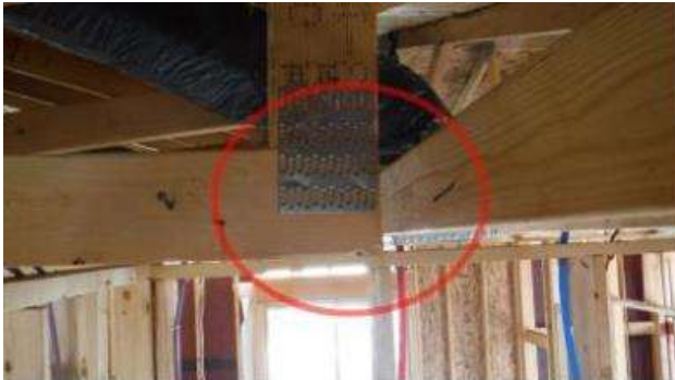
NO END BEARING-UNEVEN CEILING FRAMING.
