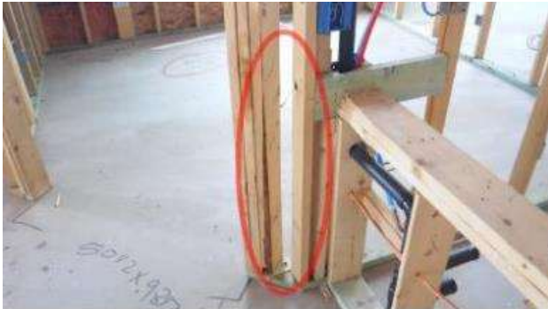
NO BLOCKING AT 45 DEGREE CORNERS / NO NAIL PROTECTION.
