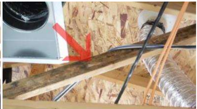
NO END BEARING-UNEVEN CEILING FRAMING / POSSIBLE MOLD AT TRUSS.
