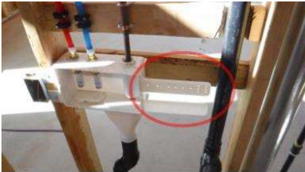
LAUNDRY BOX NOT FULLY SECURED / SUPPLY AND RETURNS CLOSE TOGETHER.
