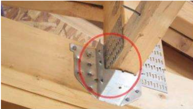
TRUSS NOT SECURED IN STRAP / SEPARATIONS AT WINDOW FRAMING.
