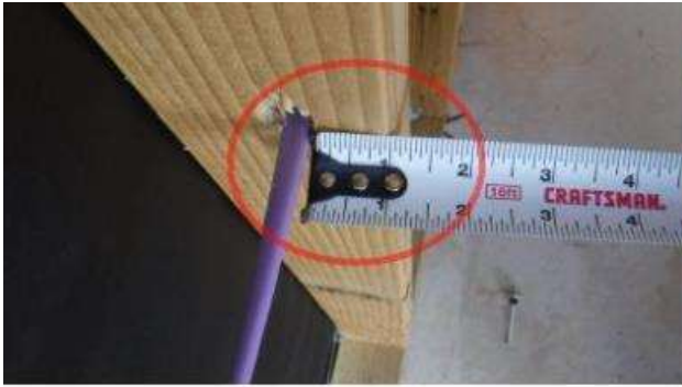
MISSING NAIL PROTECTION / POSSIBLE MOLD AT SILL.
