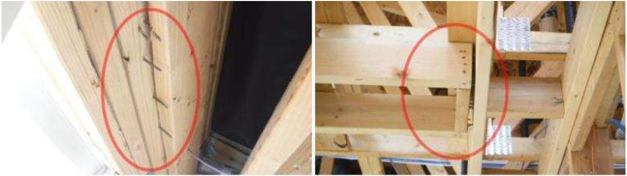
RSHINERS AT WALL FRAMING / SEPARATIONS AT TRAY CEILING.
