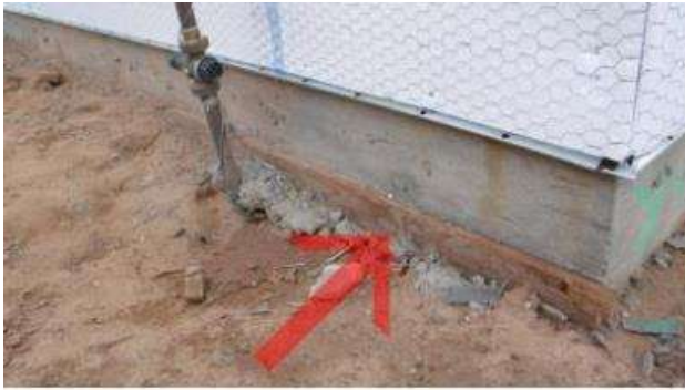
NEED TO REMOVE FORM BOARD / CHIPS IN FOUNDATION.
