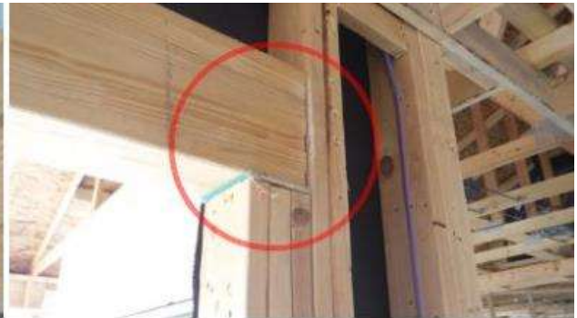
SHINERS AT WALL FRAMING / SEPARATIONS-UNEVEN FRAMING AT PATIO DOOR.
