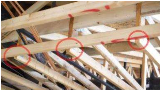
NO END BEARING-UNEVEN CEILING FRAMING / POSSIBLE MOLD AT TRUSS.
