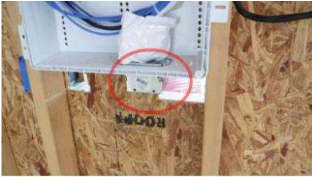
NO WIRING AT NETWORK PANEL OUTLET / LOOSE STRAP AT ENTRY.
