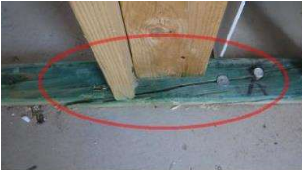
SPLIT SILL PLATE / SHINERS AT CLOSET.
