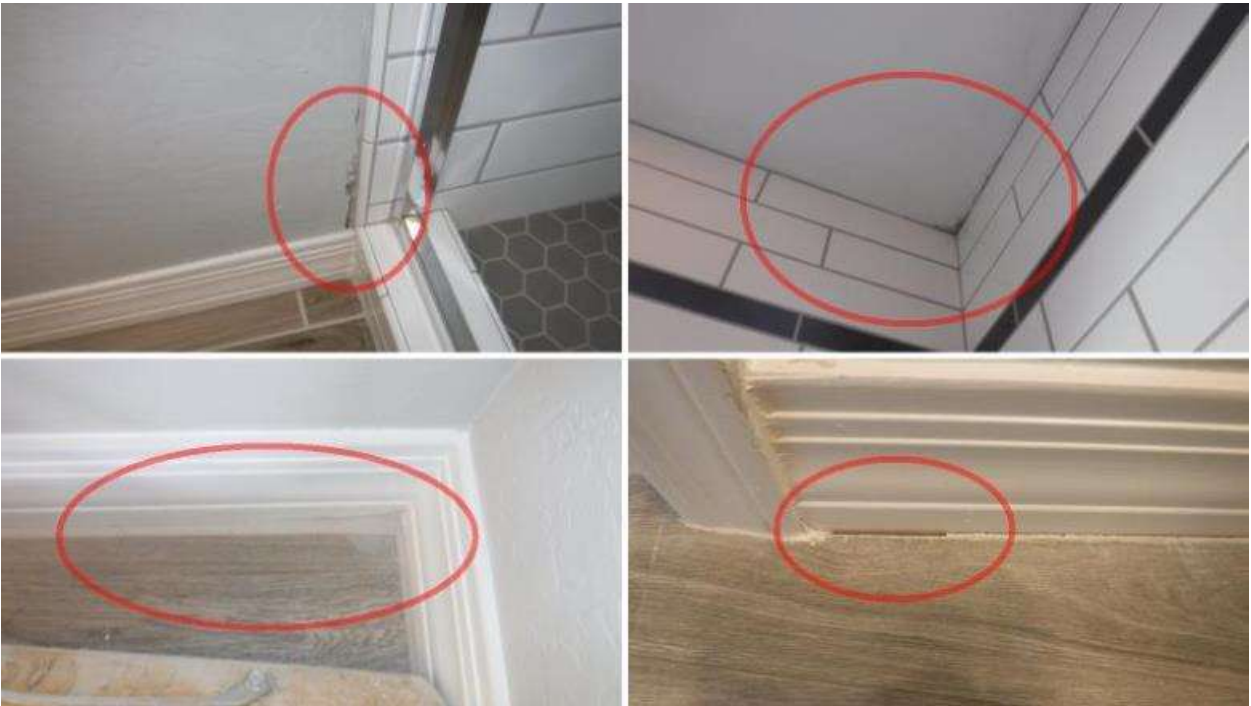
Carpet, Tile. Excessive grout line viewed near entry door. Cracks / separations in grout viewed.
