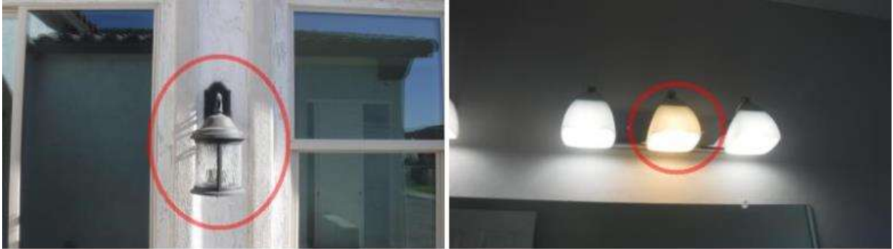
Uneven fixture; entry north between windows. Different bulbs noted; bathroom vanities.
