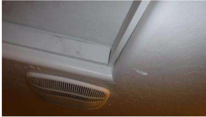
Drywall, Typical cracks noted. Uneven grout viewed; north suite above shower. Separations at attic access trim.
