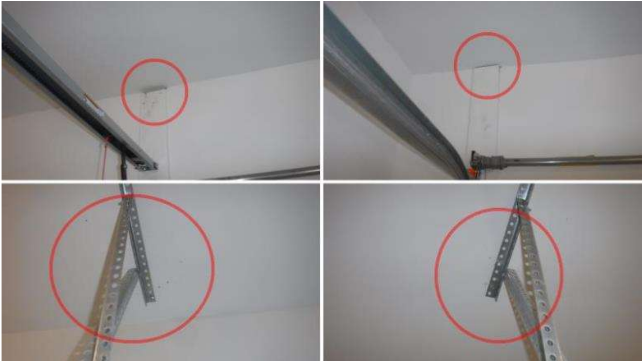
Typical cracks noted, Separations at vehicle door frame / drywall connections noted. Voids viewed near vehicle door tracks. Settlement crack viewed at ceiling near water heater. Separations at baseboards. Scuttle lid does not appear to be fire-rated, Repair any openings with approved materials to restore its fire rating. Separations at attic access trim.
