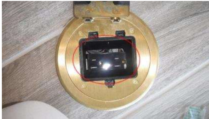
GFCI outlets are operational. Uneven floor outlet: family room northwest.
