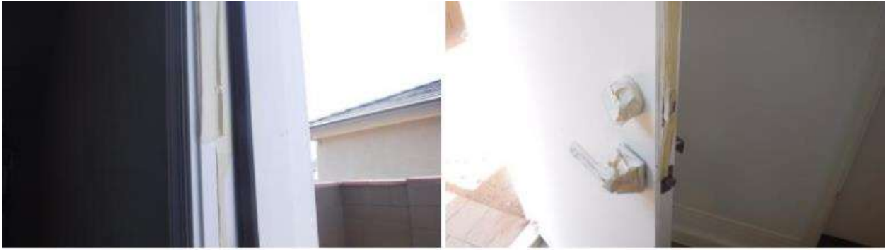
Tape / residue viewed at frame, door edge.
