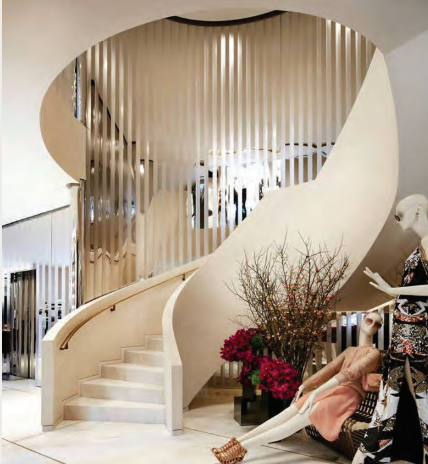
Brushed, mirrored and etched stainless steel wall cladding, steel staircase with brass handrail
