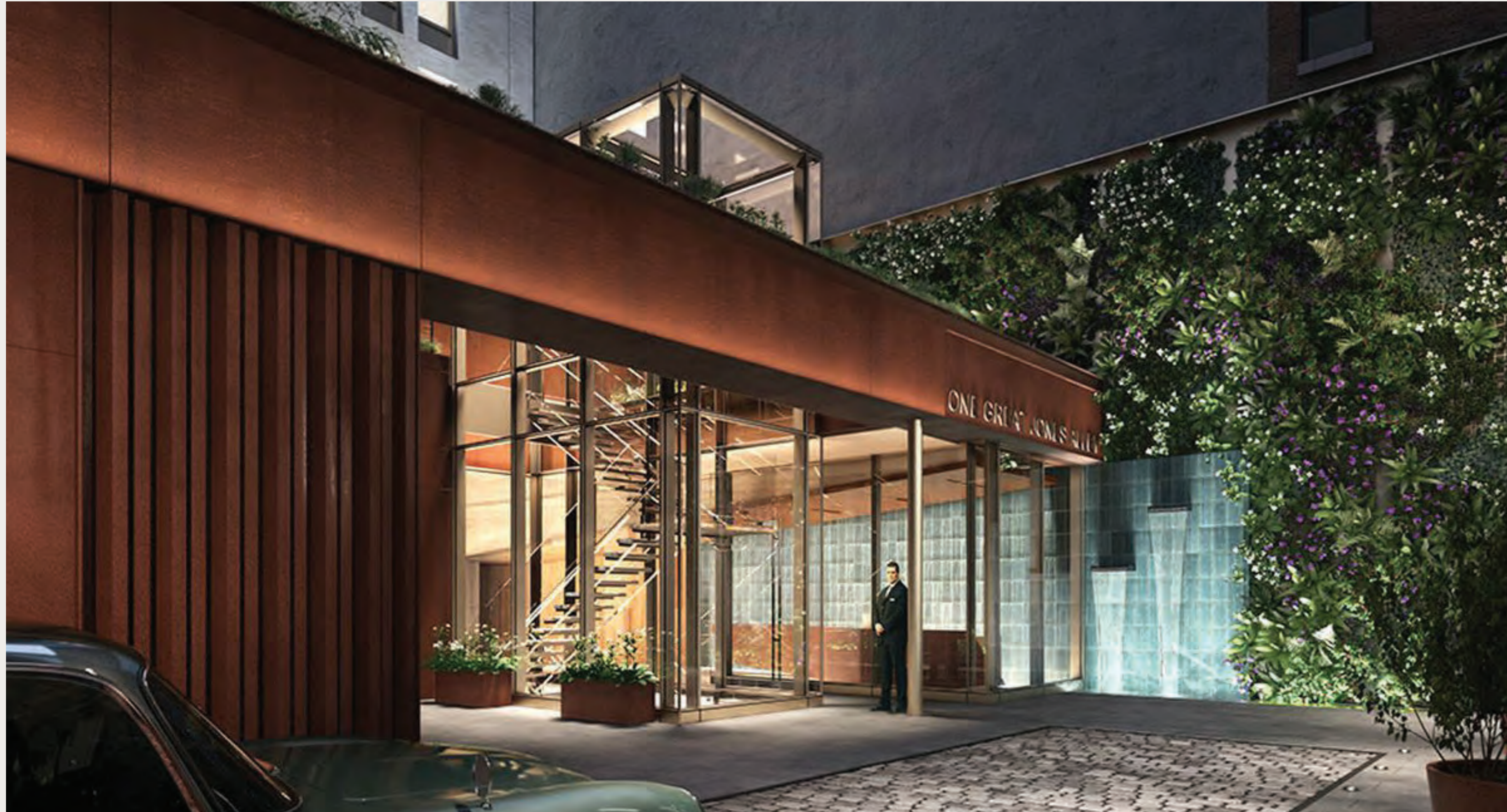
Weathered steel wall and beam cladding, louvers, signage
