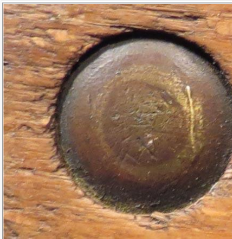
Above shows the wood swelling around the screw, some chipping is evident.
