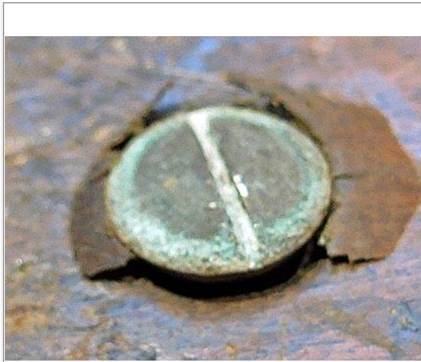
Above you can see the wood has lifted when removing the screw. Catching it at this point can help restore it.
