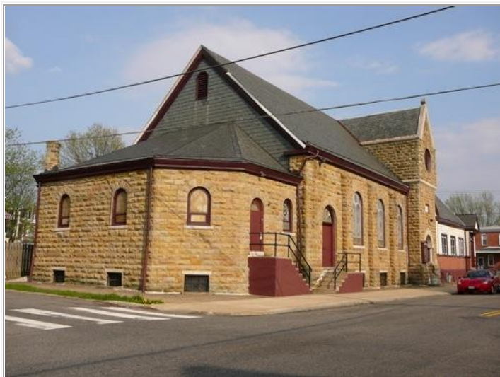
The Tacony Baptist Church is partially made from discarded grind stones from the Disston factory.
