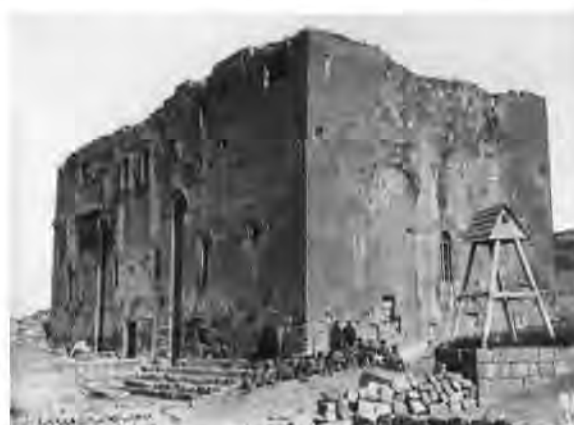
Figure 35. St All-Savior Church view from Southeast
