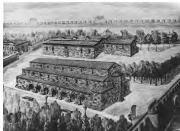
Figure 35. Central Square Reconstruction
