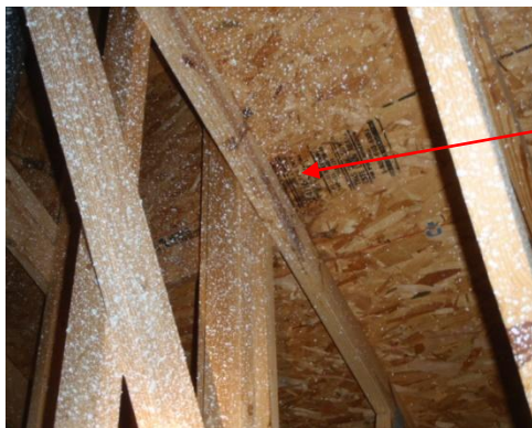
Staining on truss members
