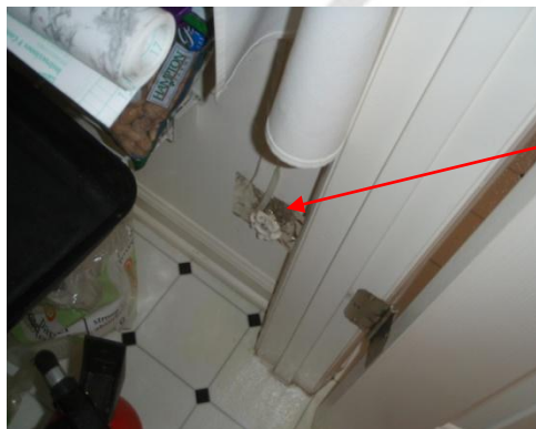
Water shut-off valve
