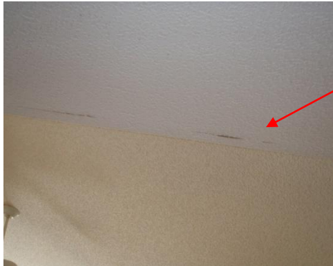
Crack kitchen front wall at living room interface
