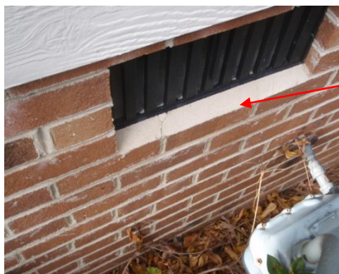
Crack right side
