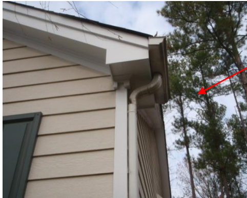
Downspout is deformed
