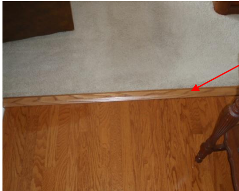
Threshold is loose
