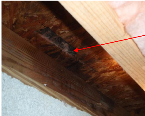
Floor under door to deck is wet
