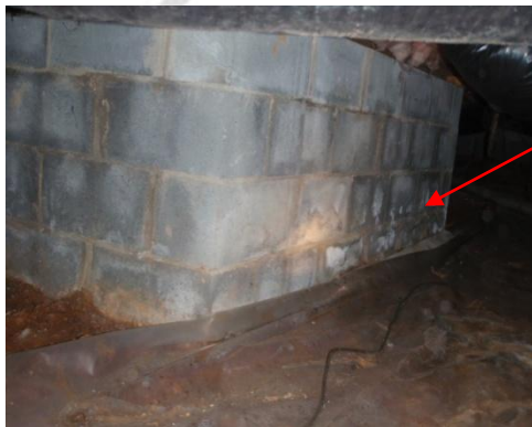
Evidence moisture came through front wall
