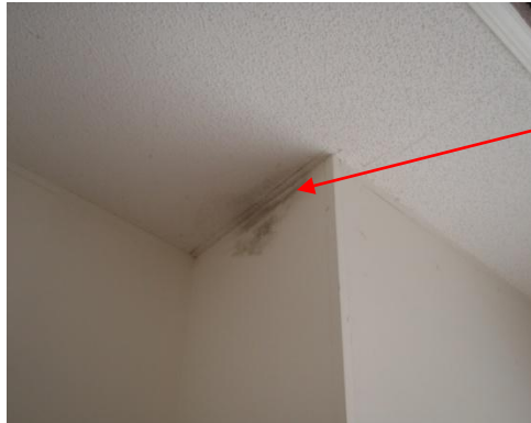
Staining on drywall
