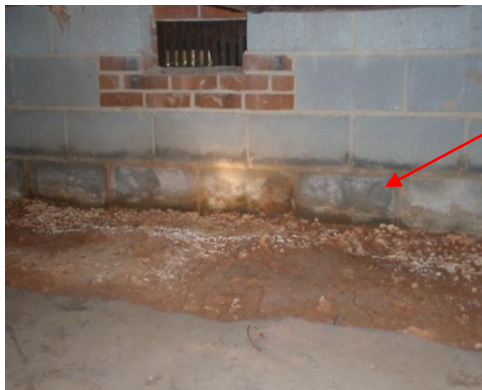
Moisture penetrating foundation wall
