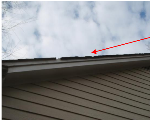
Damaged shingles on right side
