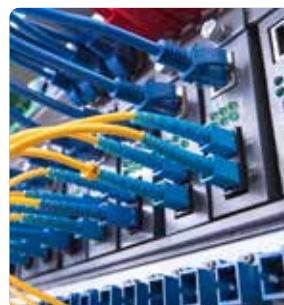
Data/Voice Cabling works
