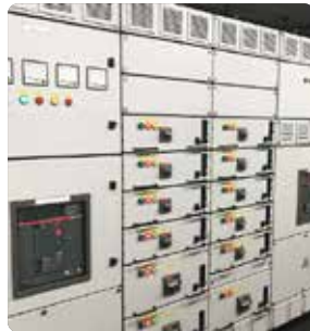
L.V Switchgear Assembly and Installation
