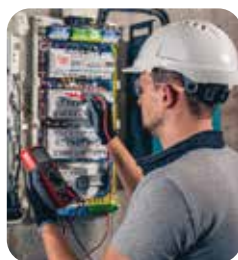
Distribution Boards HV&MV
