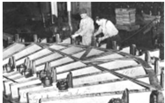
Jigs for clamping and curing laminates
