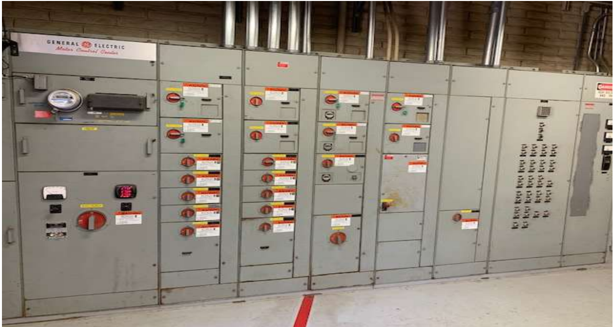
Electrical Point of Interconnection
