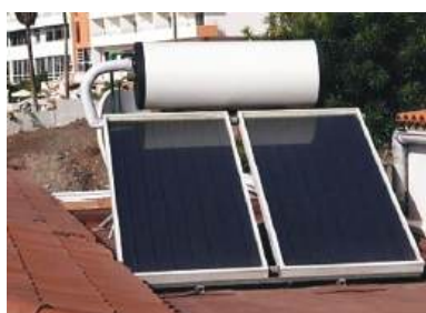
Fig. 12.3 Solar flat plate collector
