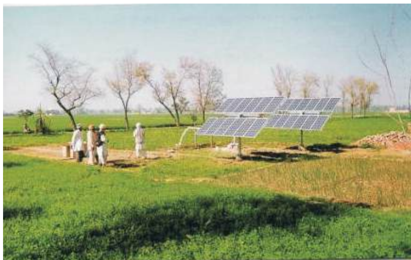
Fig. 12.2 Photovoltaic Water Pumping
