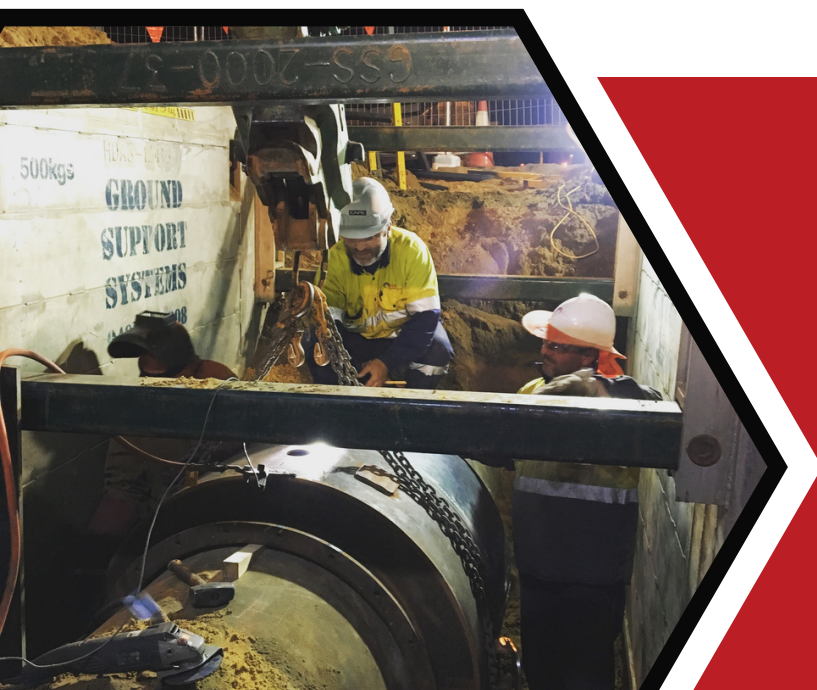
Burst water main convex band repair
