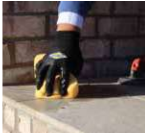
PIC 2. Remove excess grout with clean water.
