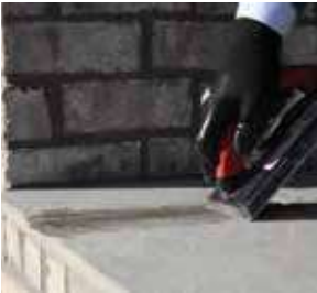
PIC 1. Fill joint with grout.
