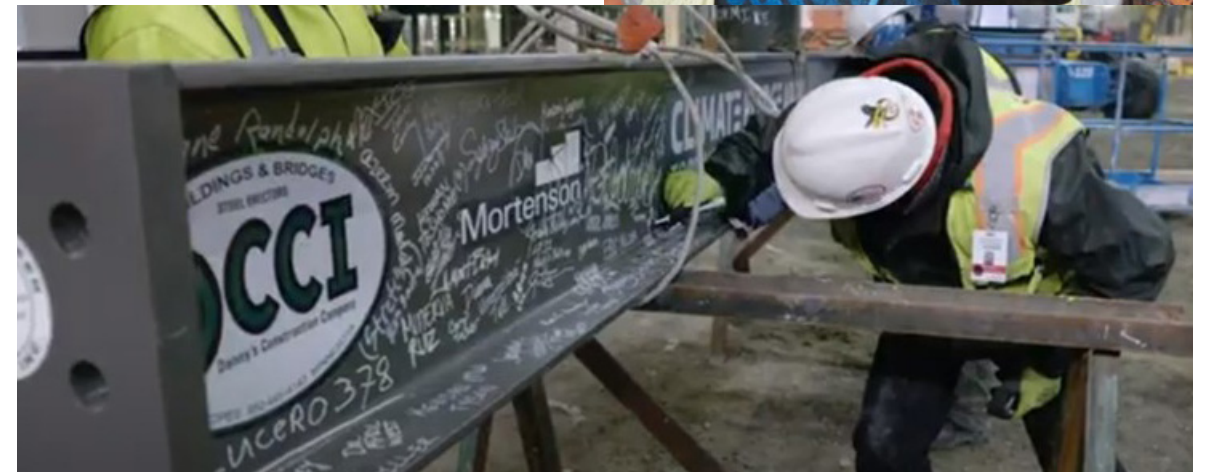
Workers celebrate completion of structural steelwork on the Arena by signing a beam. Photo courtesy of Climate Pledge Arena's YouTube channel.
