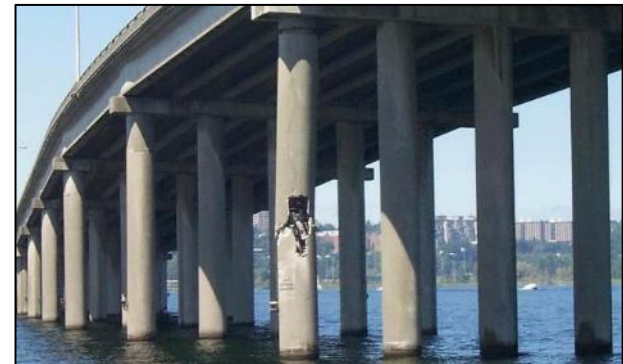
Photo of old, hollow concrete columns for original SR 520 bridge structure.
