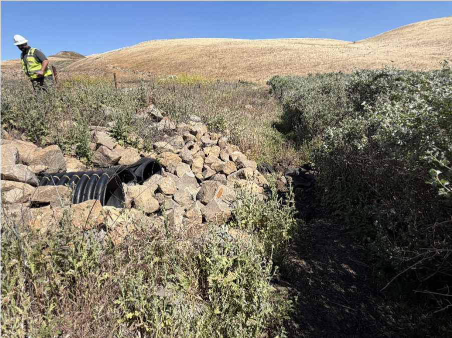
Photo 5. Erosion restoration at the Mitigation Pond
