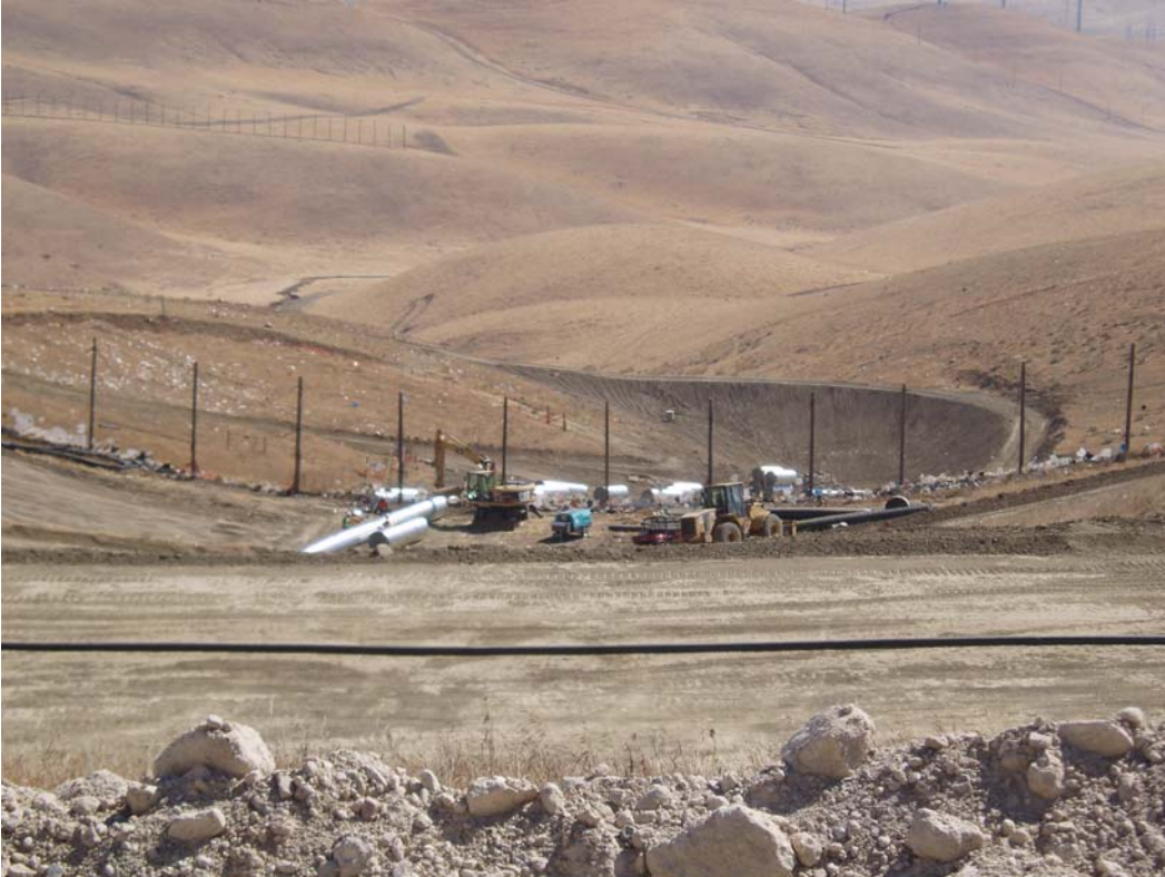
Drainage and Culvert Repair Viewed from Above, Looking East – September 8, 2008
