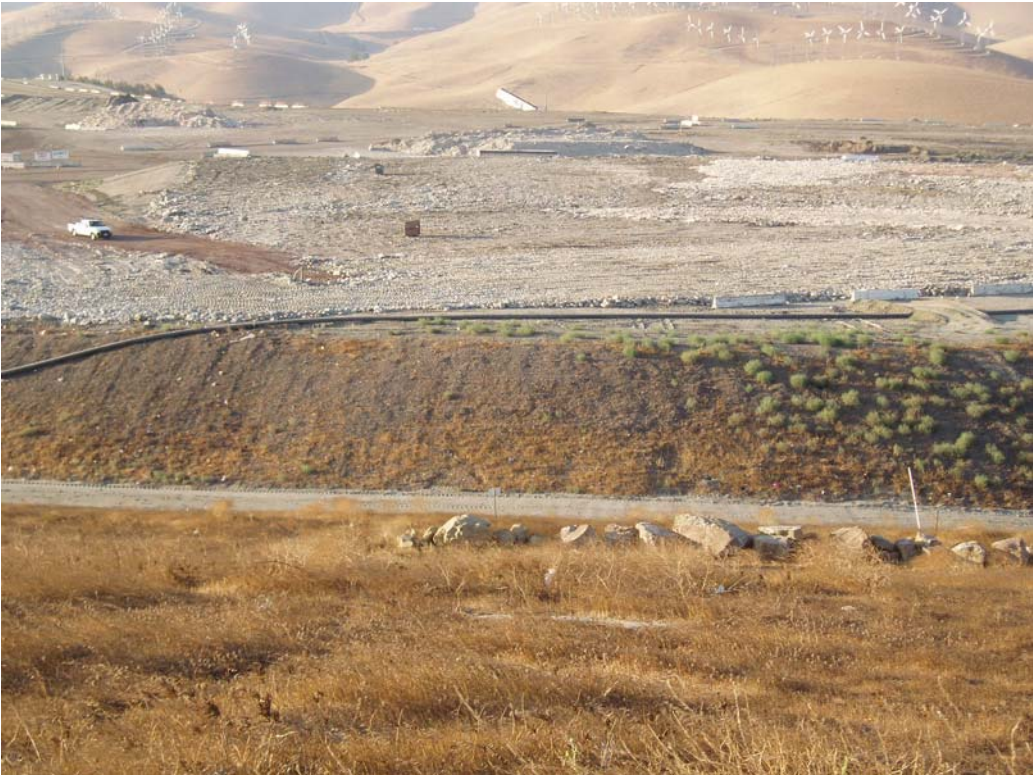
Winter Pad Preparation, Looking South – August 15, 2008
