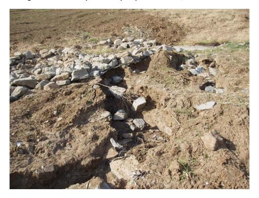
Figure 1 – Erosion problem upslope of Basin B, November 2008
