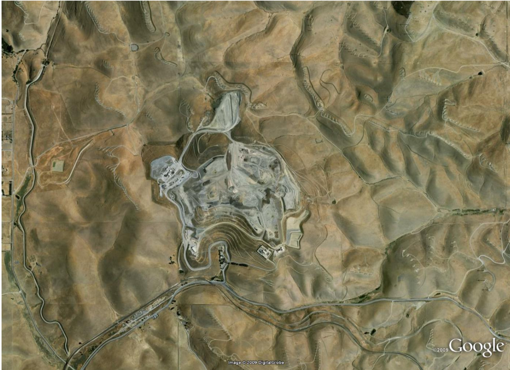
Figure 1 - ALRRF aerial view, 2008
