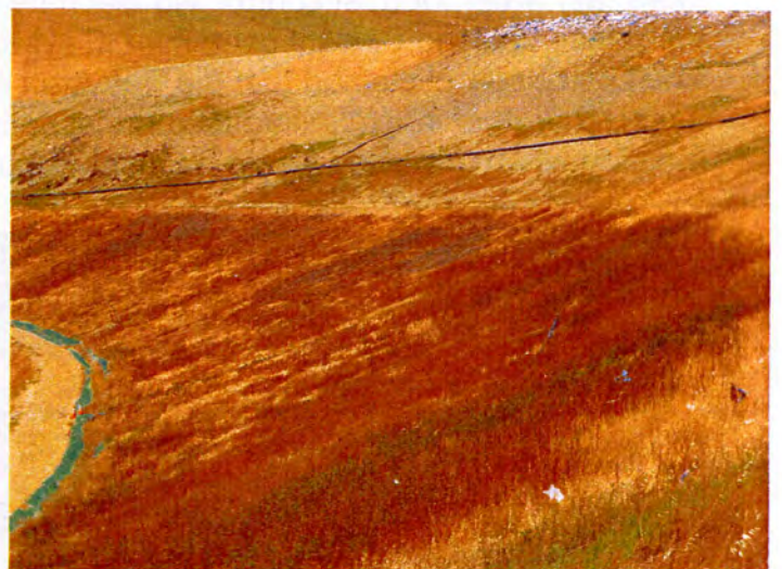
The first photograph shows the screen material that was installed in the runoff ditches as a method for controlling sediment running off the landfill. The presence of sediment in the trough indicates that additional controls are needed to control sediment runoff. The second photograph shows dead vegetation on the landfill slope. Improving the vegetation on the southern slope of the landfill should be part of the landfill's winterization program for the upcoming wet season.
