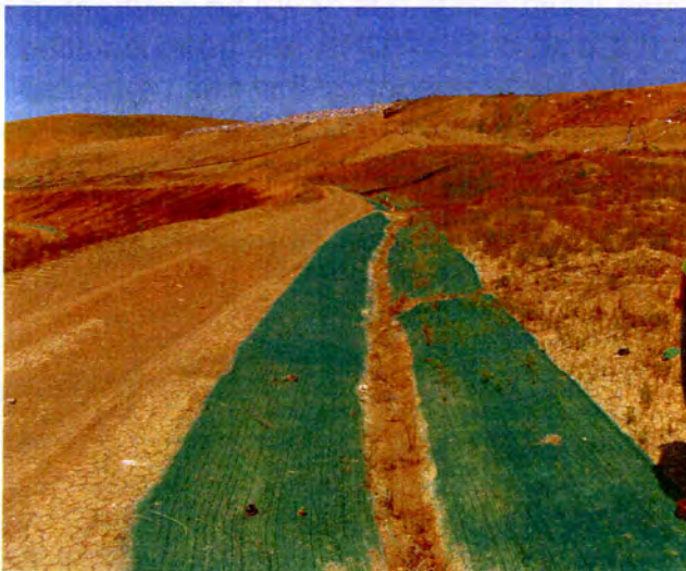
The first photograph shows the screen material that was installed in the runoff ditches as a method for controlling sediment running off the landfill. The presence of sediment in the trough indicates that additional controls are needed to control sediment runoff. The second photograph shows dead vegetation on the landfill slope. Improving the vegetation on the southern slope of the landfill should be part of the landfill's winterization program for the upcoming wet season.
