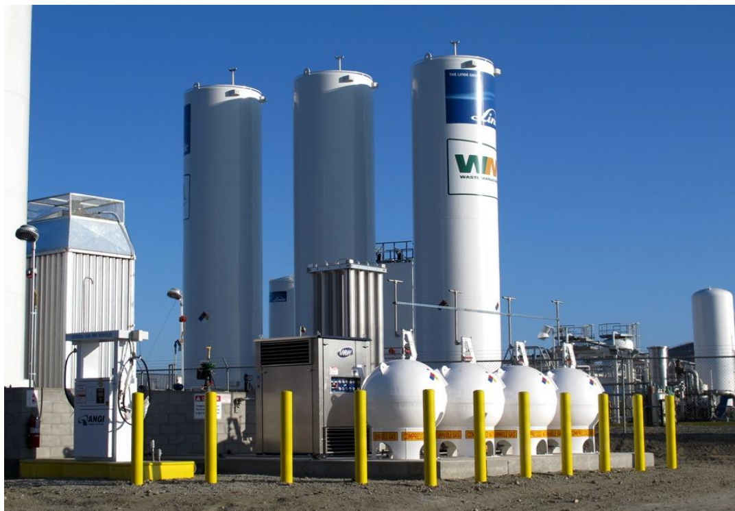
Fueling facility is in foreground, surrounded by yellow bollards. Tall structures are part of existing LNG plant.
