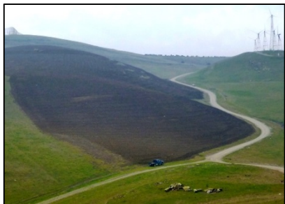
Fill Area 2, to be excavated prior to receiving waste.
