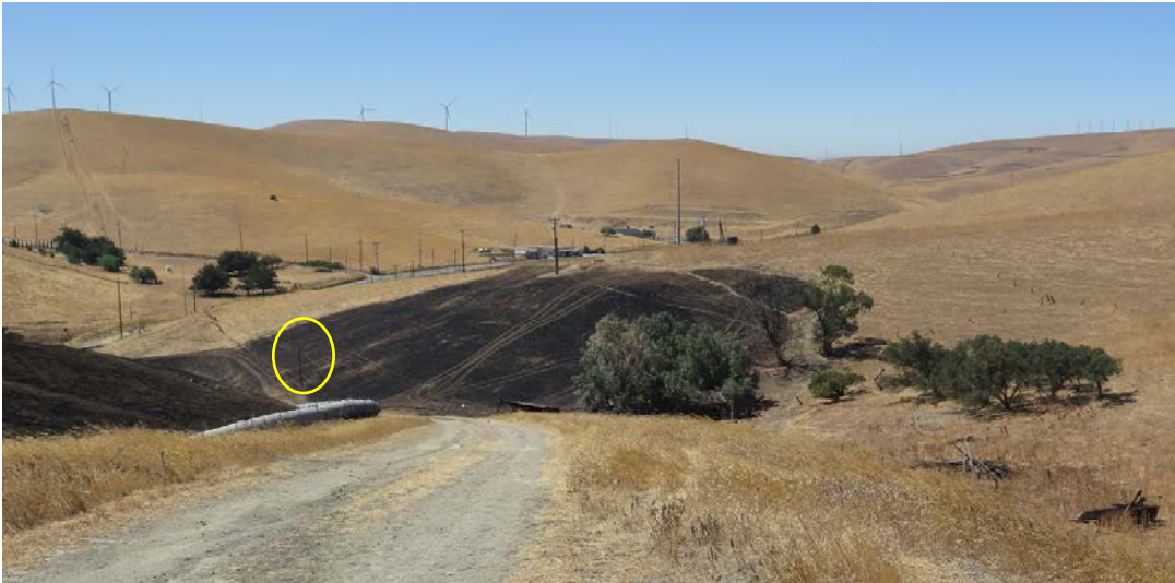
Upper portion of access road to Basin C; note metal drain pipe on the left. Looking SSW. Fire apparently originated at utility pole inside yellow ellipse.
