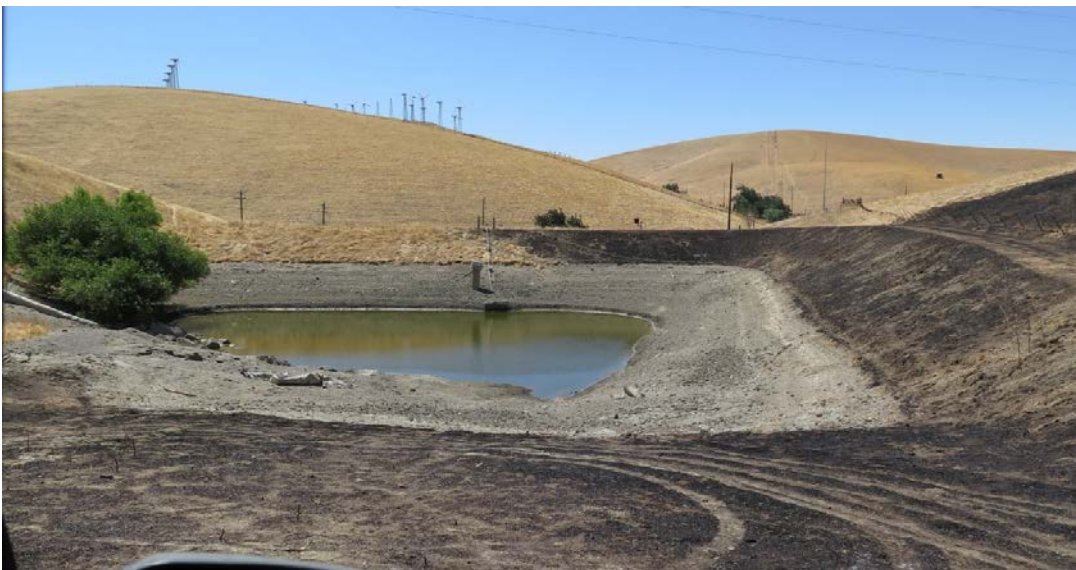
Basin C, looking south.
