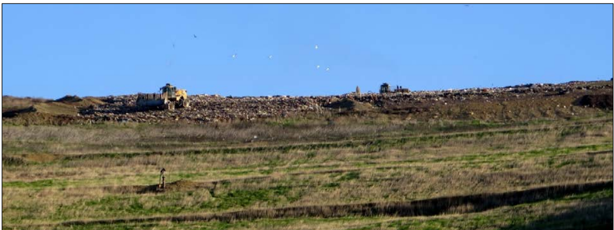
Steep portion of ET cover area, viewed from below
