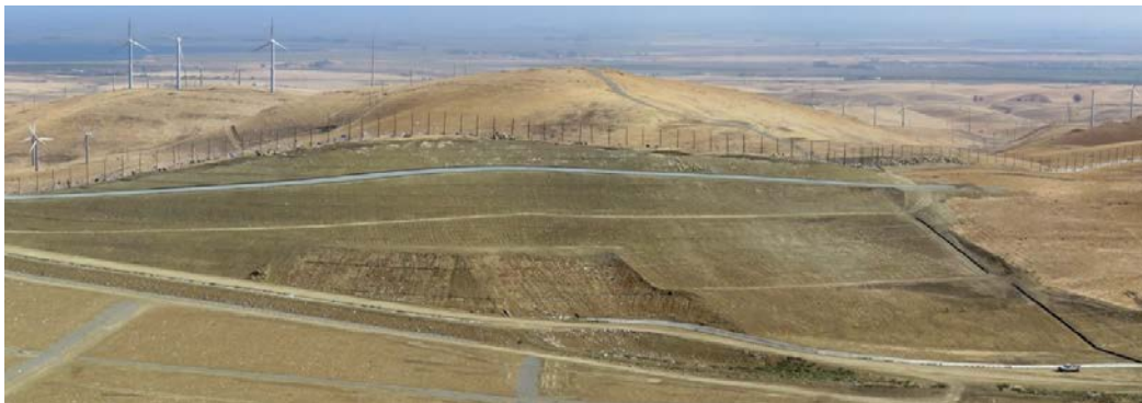
Phase 2 excavation, with wattle, benches and downdrain in place.
