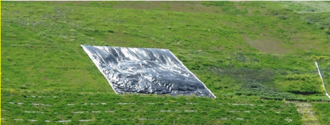
Landslide Above Fill Area 2, Phase 1
