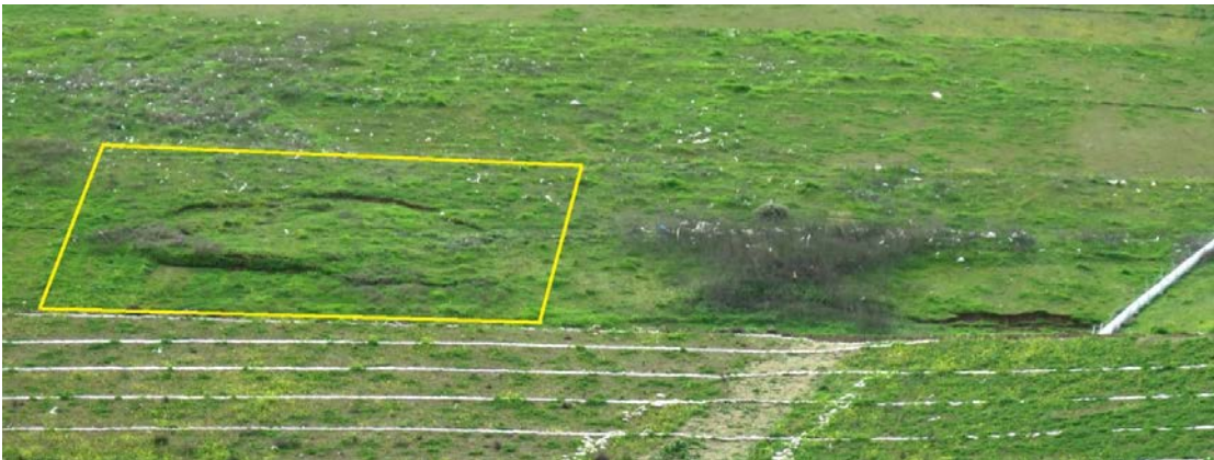
Landslide Forming above Fill Area 2, Phase 1
