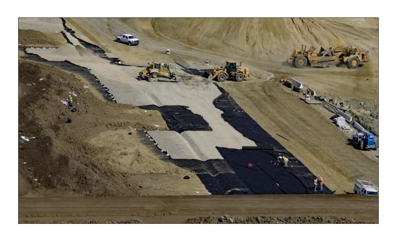
The photo on the cover of this report shows construction of the liner for the Phase 2/2B portion of Fill Area 2, viewed from the hill immediately to the west. The photo was taken on October 11, 2019.
