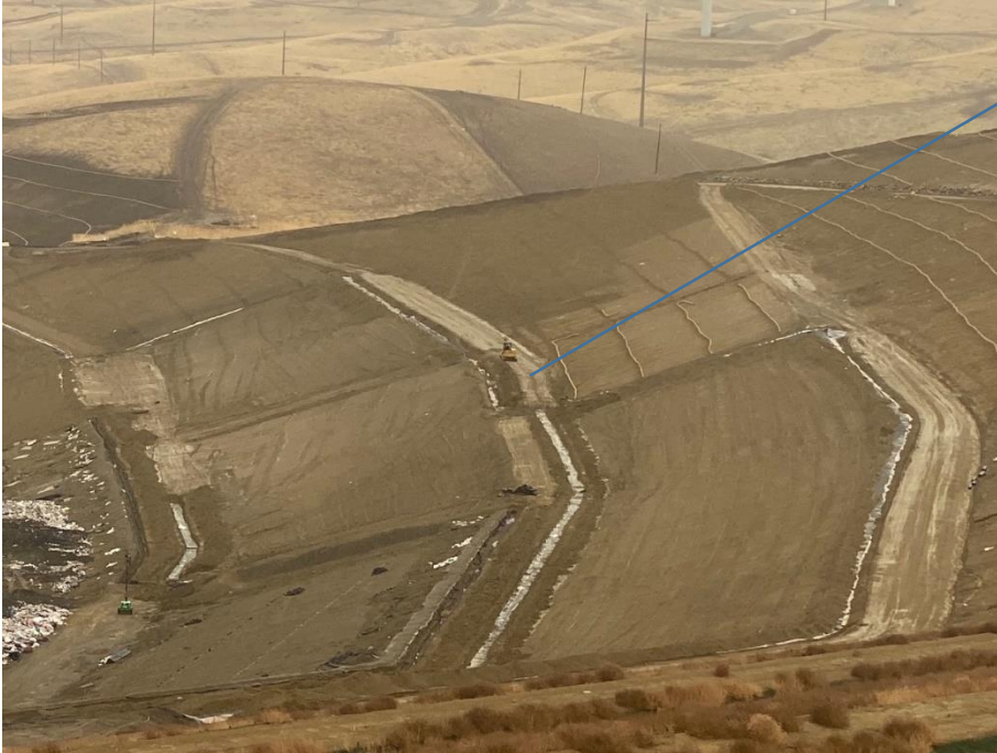
Compaction at Phase 5 construction
