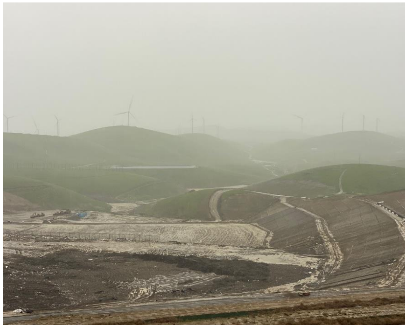
Grading on FA2, Phase 5 by SUKUT
