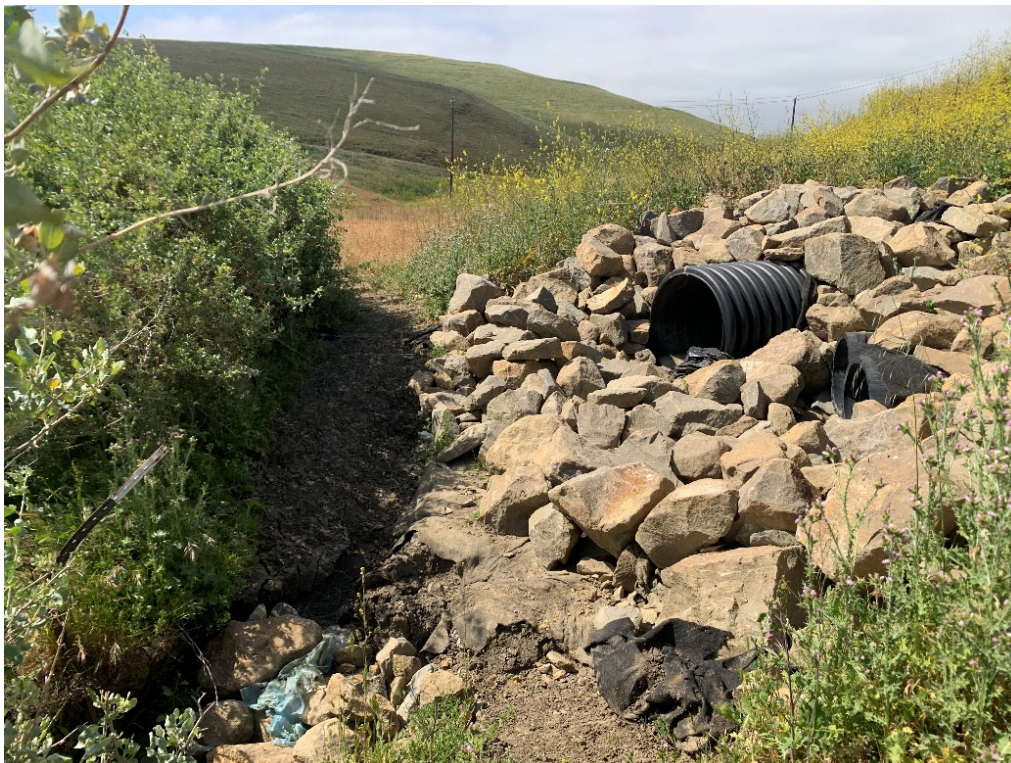
Photo 7. Restored culvert outfall west of mitigation pond
