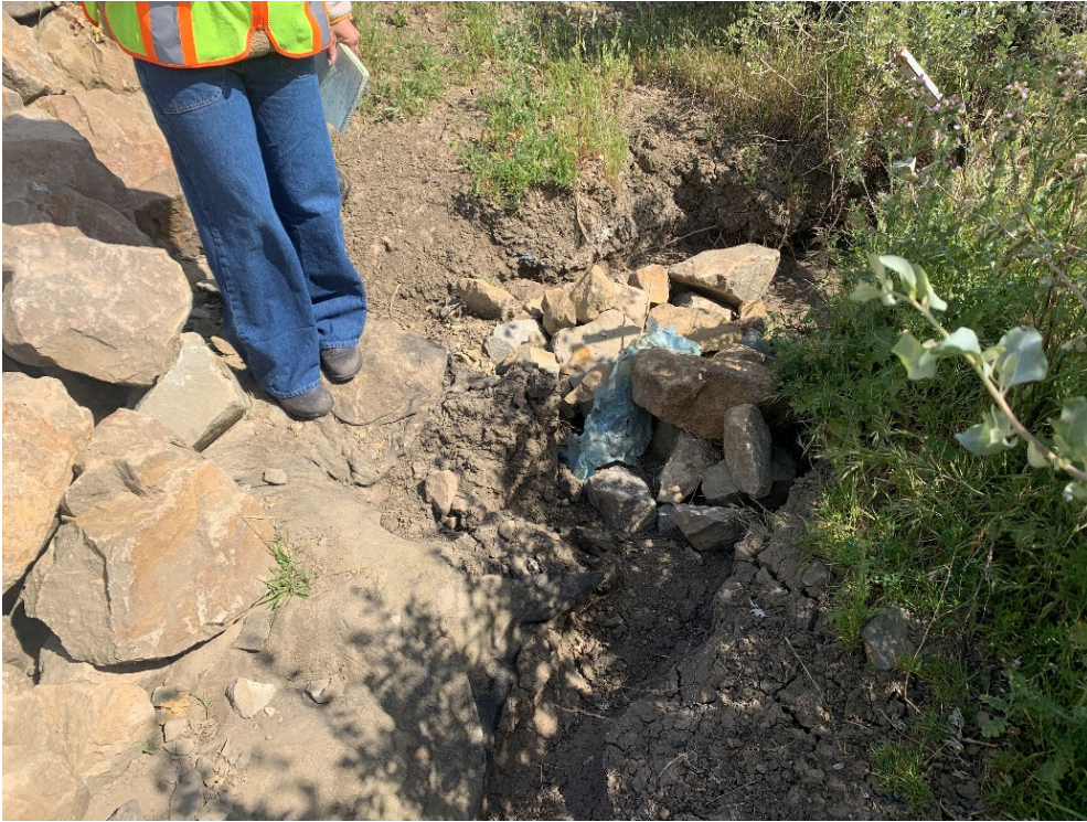
Photo 8. Erosion at restored culvert outfall west of mitigation pond
