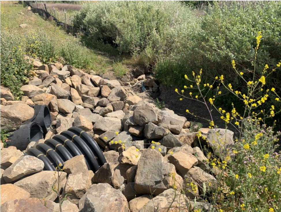
Photo 6. Erosion restoration at the Mitigation Pond
