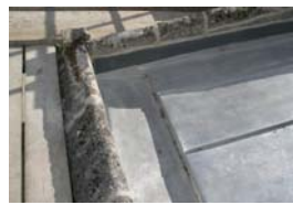
Repaired Parapet Corner Stonework
