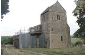
Scaffolding being erected
