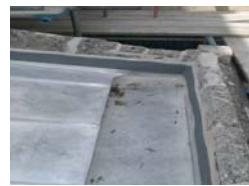
Repaired Parapet Corner Stonework
