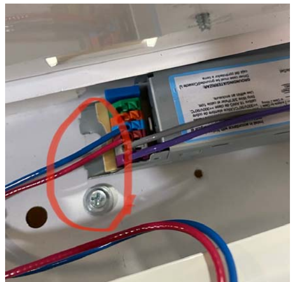
Strip light driver not installed properly, mounting screw not engaged with driver
